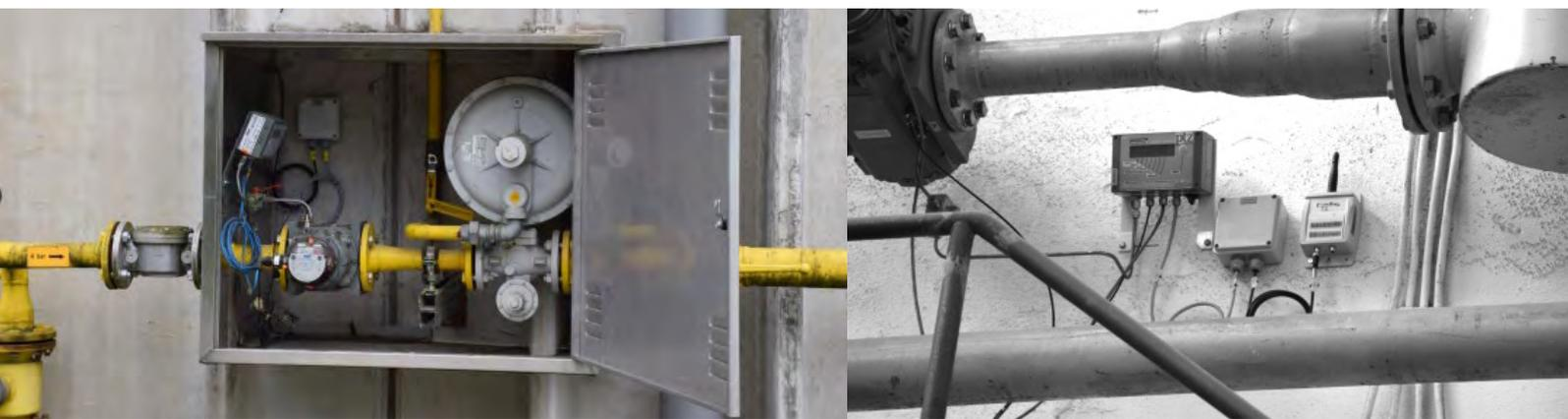
• Compressed air consumption metering using LoRaWAN communication:
