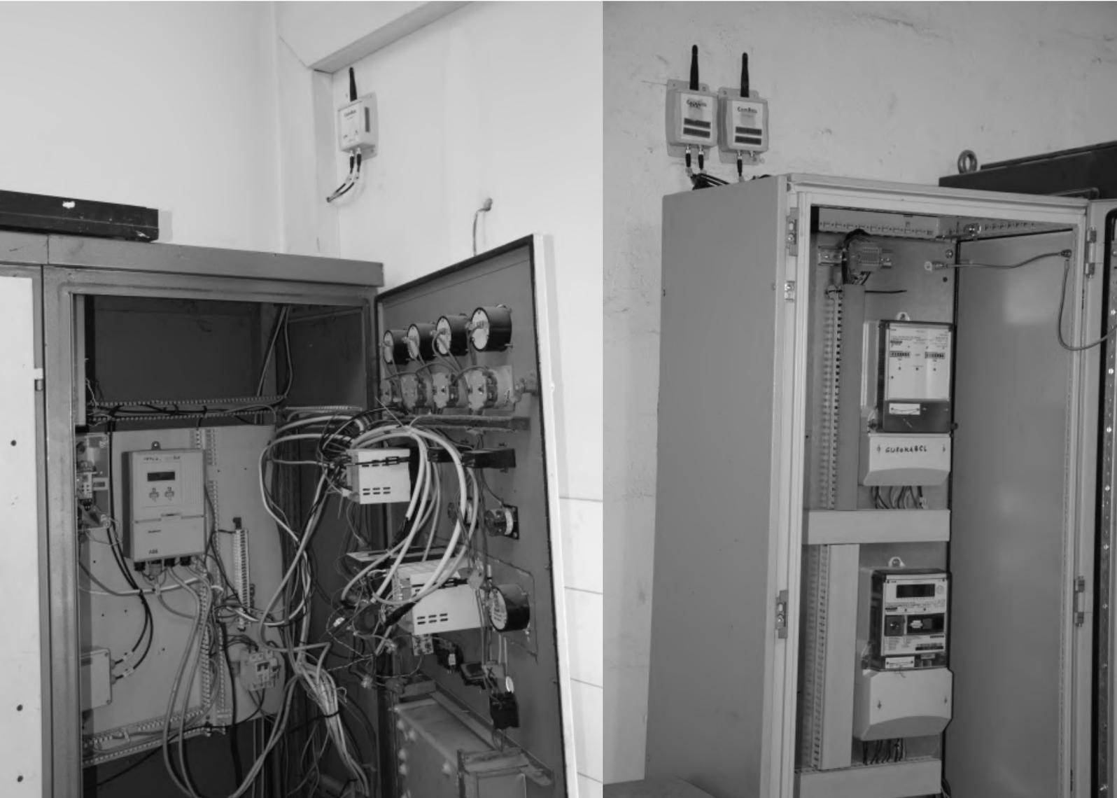
Combox.L communication devices collect data from meters in regular 15-minute intervals and transmit the readings via the “LoRa” network to gateways, which then transmit them to the EMS (Energy management system). This is all done using the standard LoRaWAN communication protocol.
